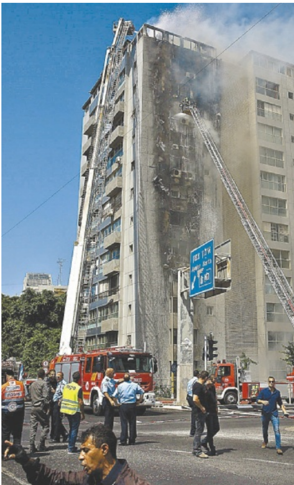
FIRE HITS RAMAT GAN HIGH-RISE: A fire engulfed the top 10 floors of a Ramat Gan residential tower near the Ayalon Highway yesterday. Police said there were no injuries but the blaze in Bialik Street led to traffic lanes being shut on the Ayalon. Tomer Appelbaum
